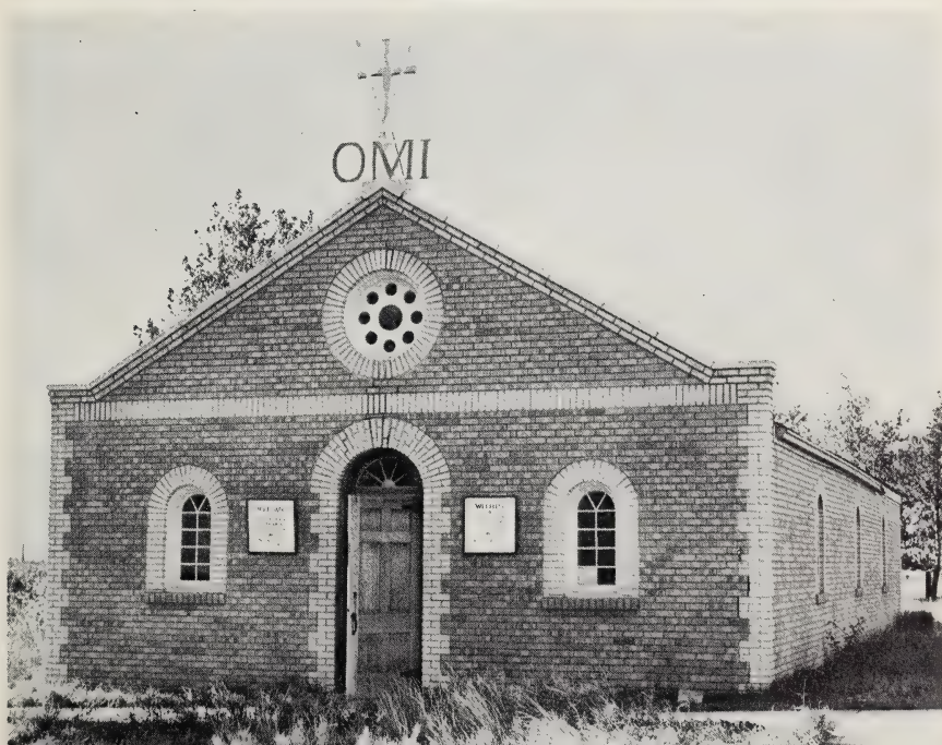
Exterior of the old log church at St. Albert is protected by a modern brick structure.
